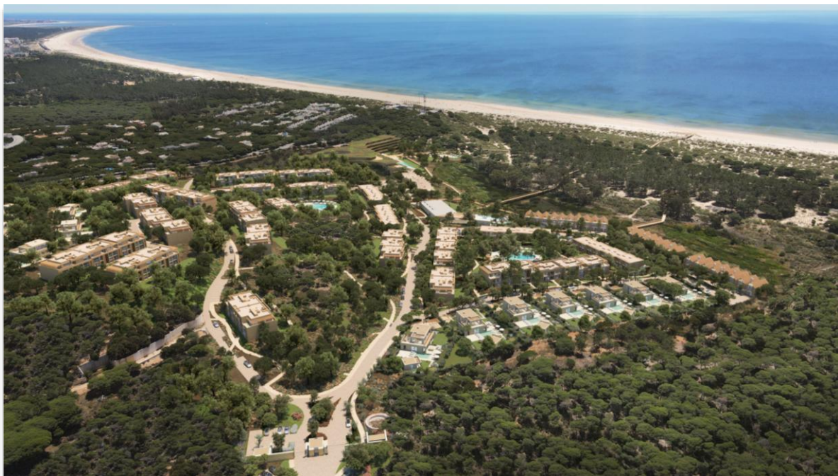
Figure 2. CGI image of Verdelago Resort at the end of construction.
